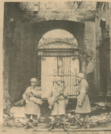
Chilean soldiers in front of bombed out Allende palace last September.
